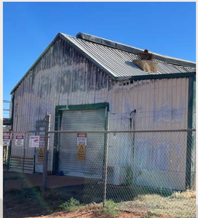
Replacement of this temporary power station to a hybrid solution is underway.
